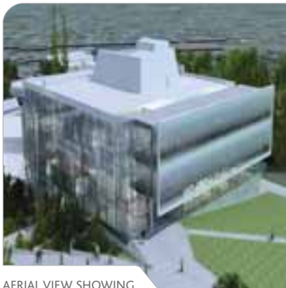
AERIAL VIEW SHOWING SOUTH/WEST FACADE
