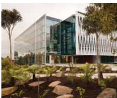
AWARD-WINNING BUILDING: The University of Waikato's new Student Centre.
